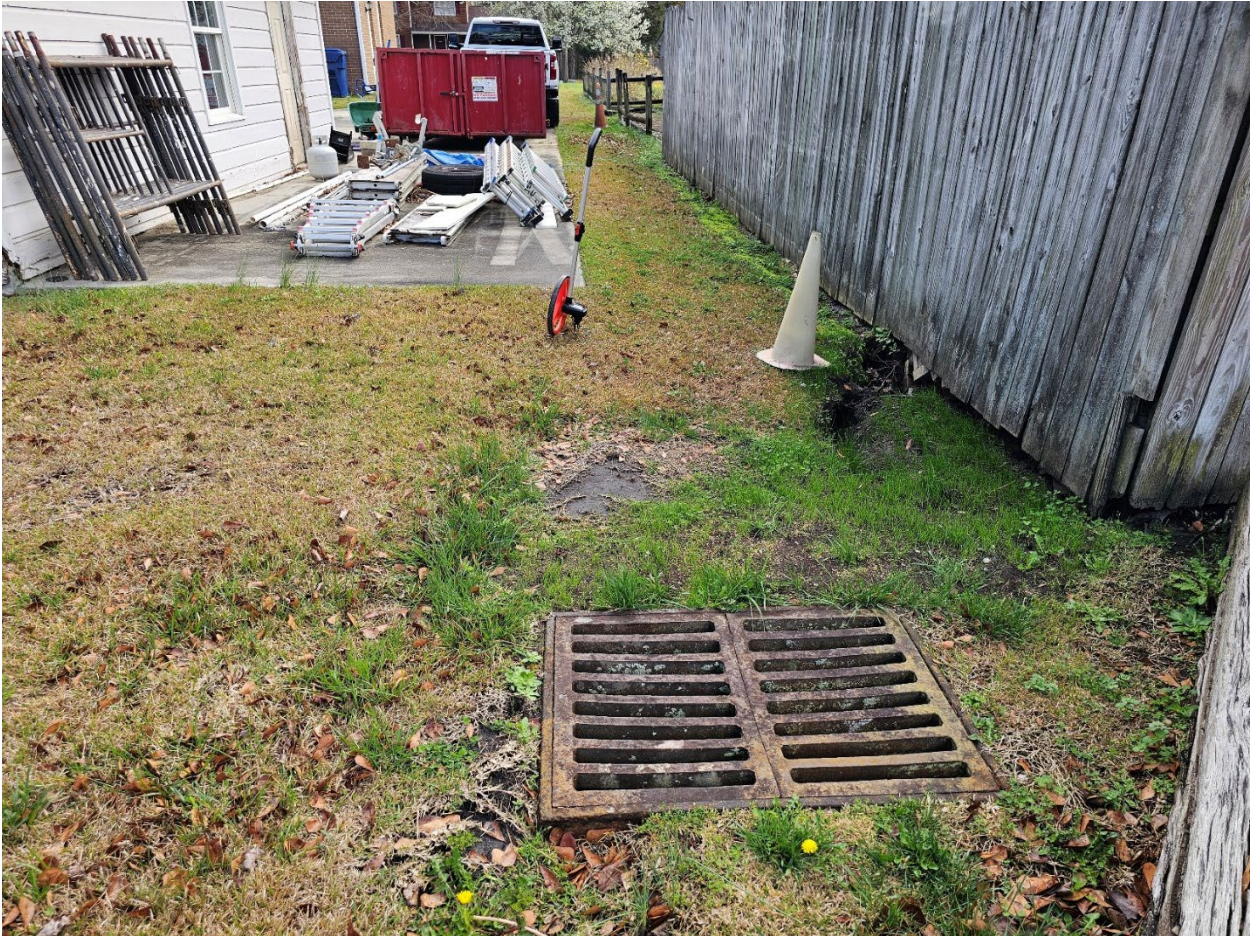
Figure 4: Catch Basin between 105 and 107 Foxhall Street
