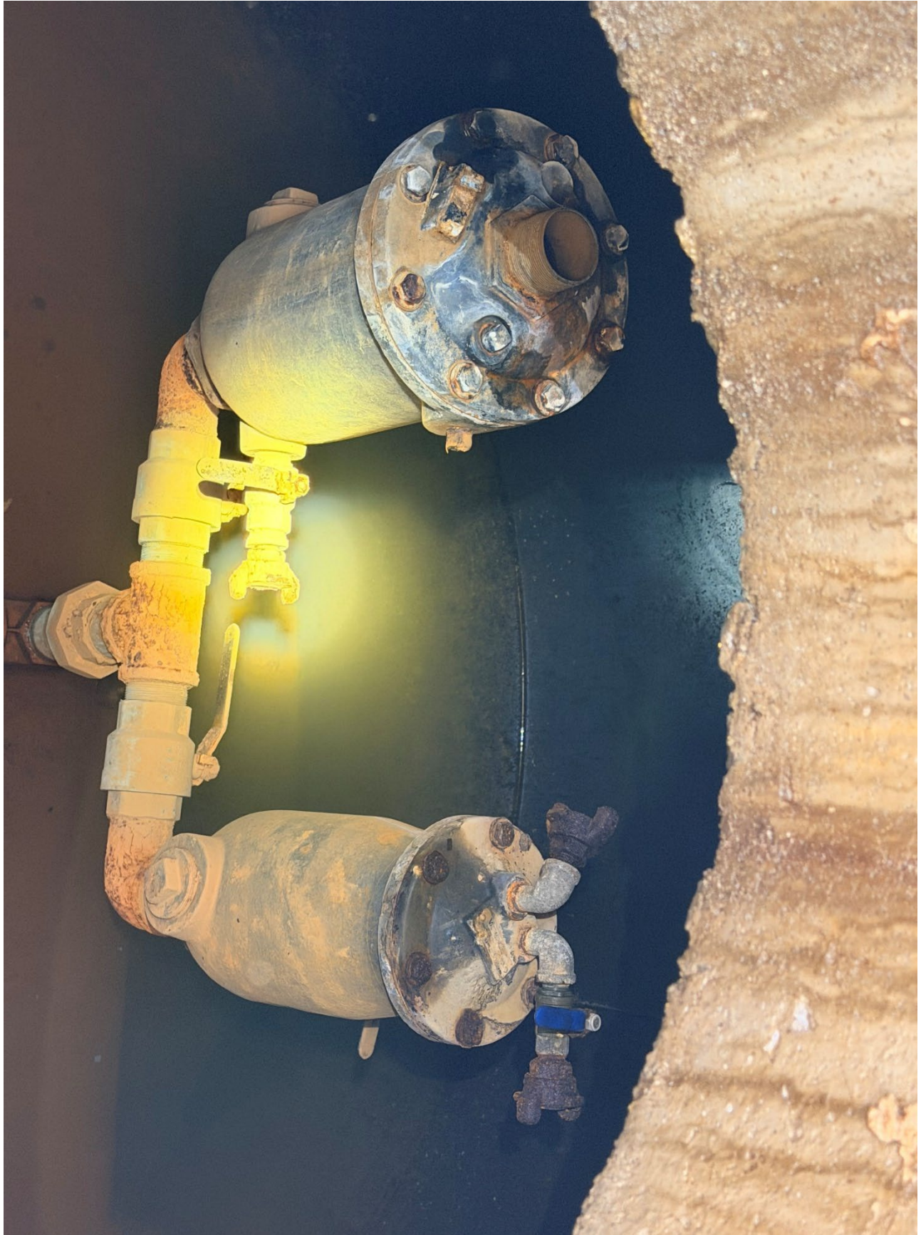
Figure 7: Val-Matic Air-Vacuum Combination Valves
