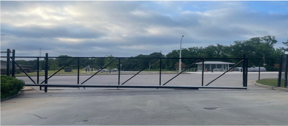
Existing Entrance Gate (45')
