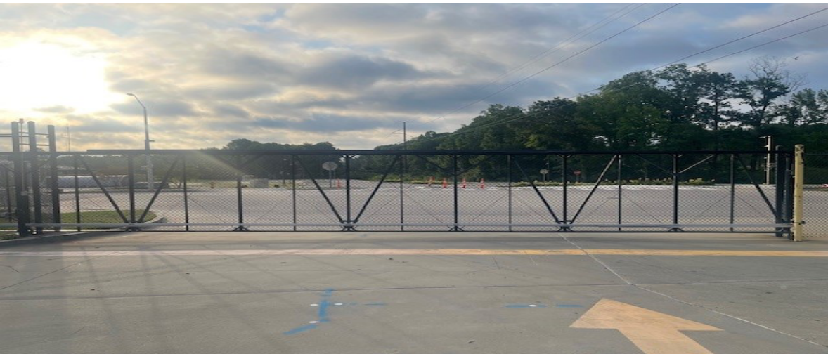
Existing Exit Gate (65')
