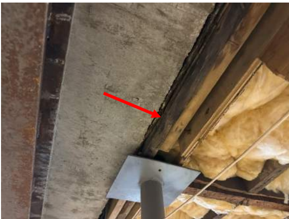
Picture 5 – Example of partially sistered, deteriorated rim band
