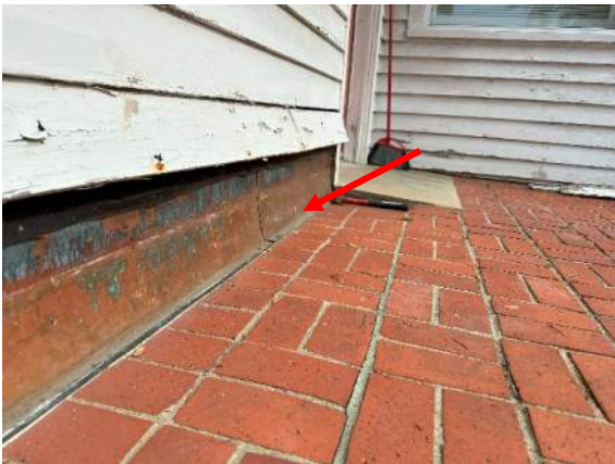
Picture 9 – Example of existing flashing at right side of patio
