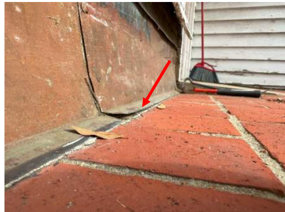
Picture 10 – Example of existing flashing at right side of patio
