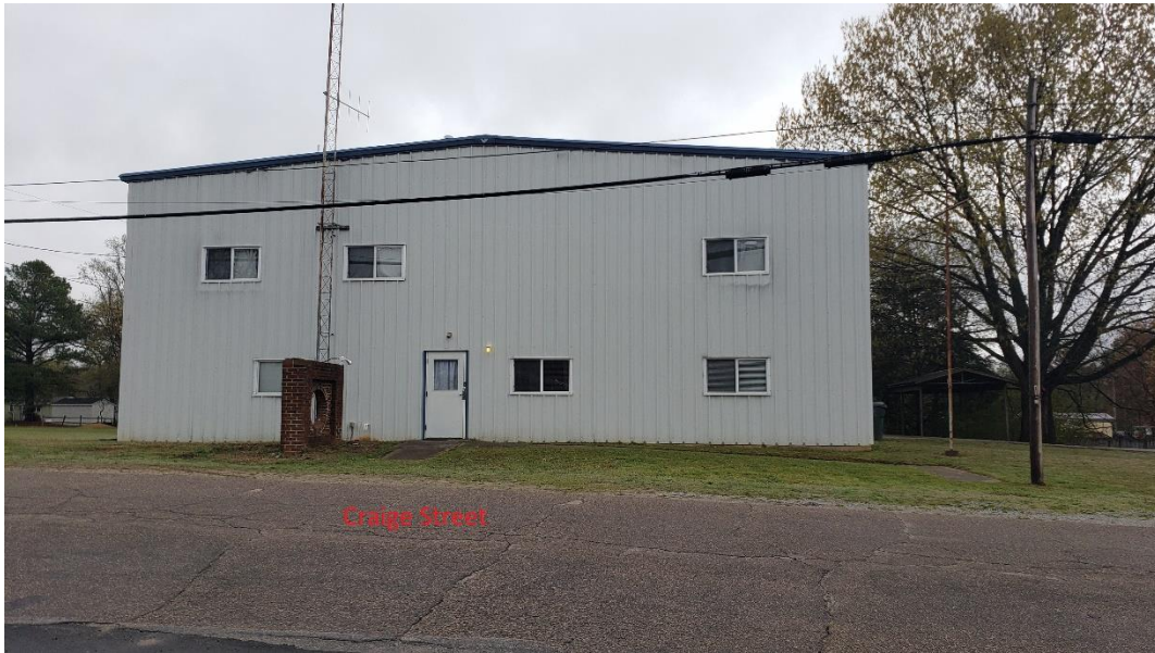
West Side Exterior
