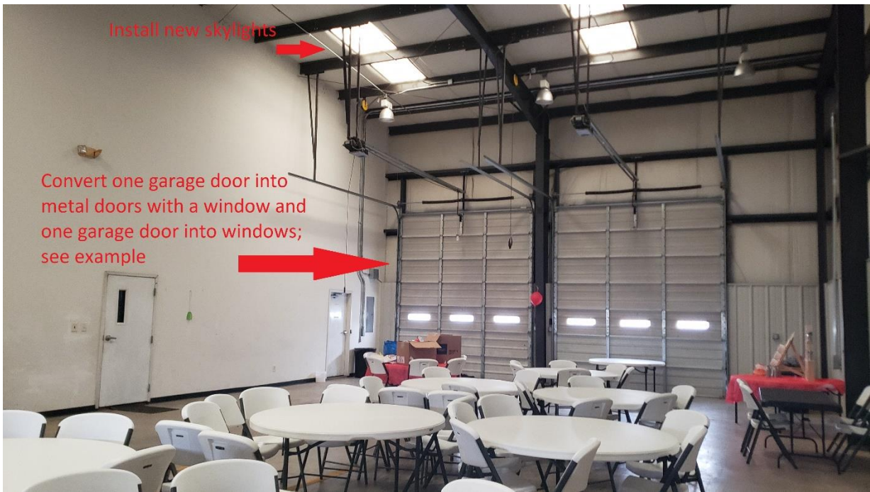
Interior Former Ambulance Bay
