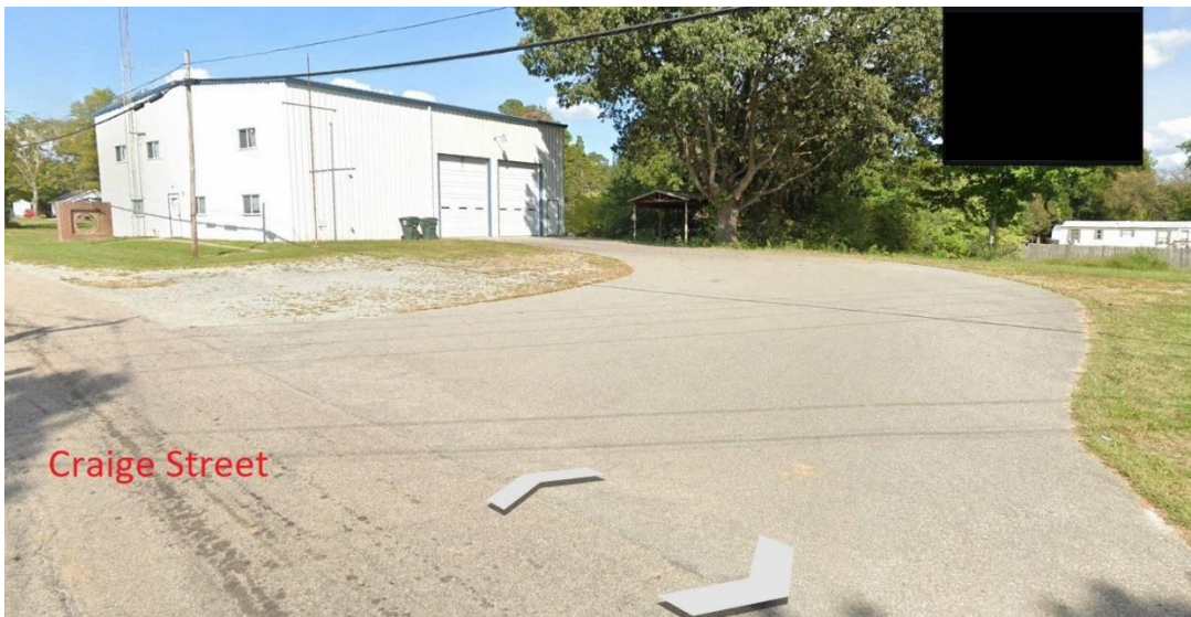
SW Corner Exterior / Existing Driveway
