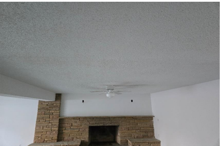
5. Basement Texture Ceiling. Sample A-10
