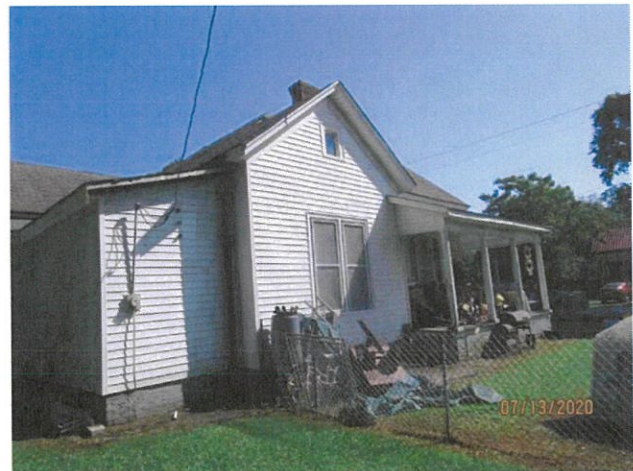
Exterior windows severely damaged.
