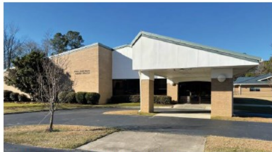
BUILDING 20 - LYNN G. KING ALLIED HEALTH BUILDING
