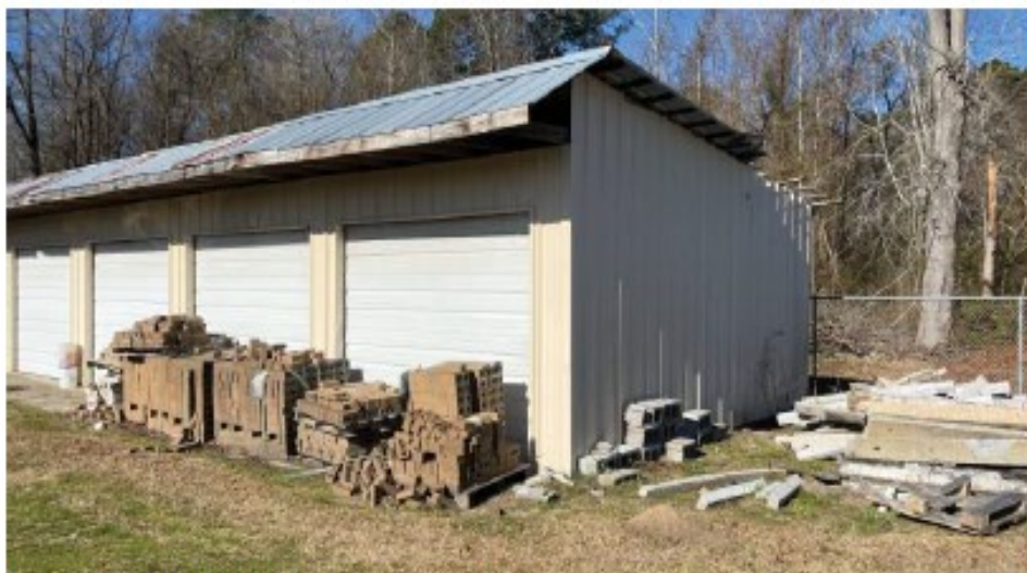
BUILDING 19 - MAINTENANCE / STORAGE
