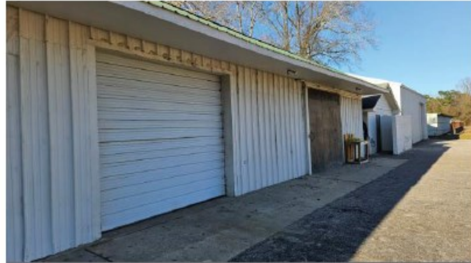
BUILDING 5 - MAINTENANCE BUILDING
