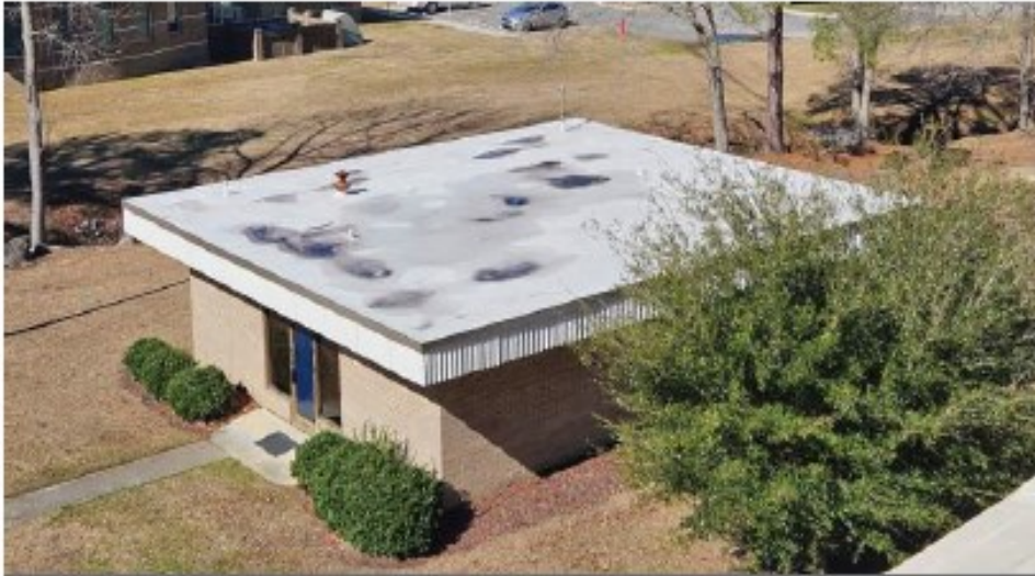
BUILDING 4 - FACILITIES BUILDING
