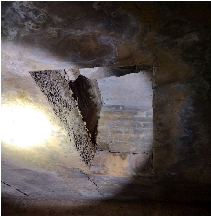
Figure 13. Opening in top slab of Bloodworth box
