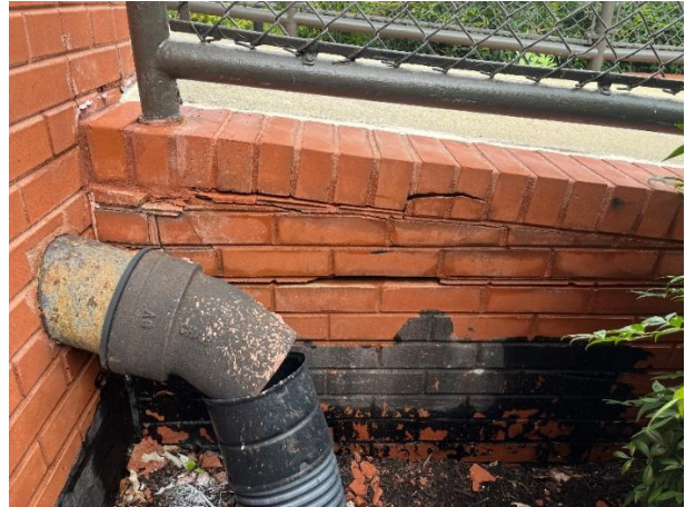
Photo 3 – Roof Drain and South Ramp Wall
