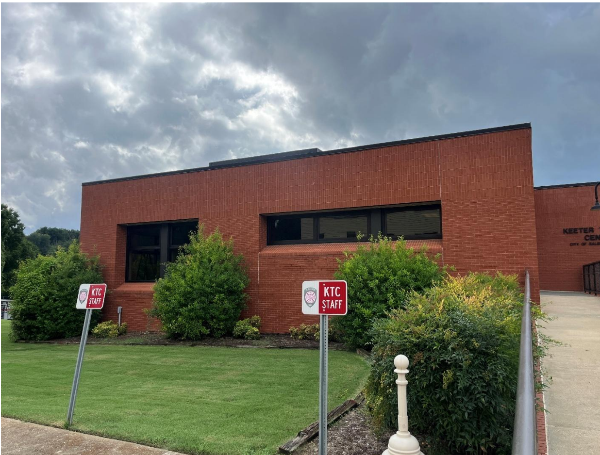
Photo 1 – Building East Elevation
