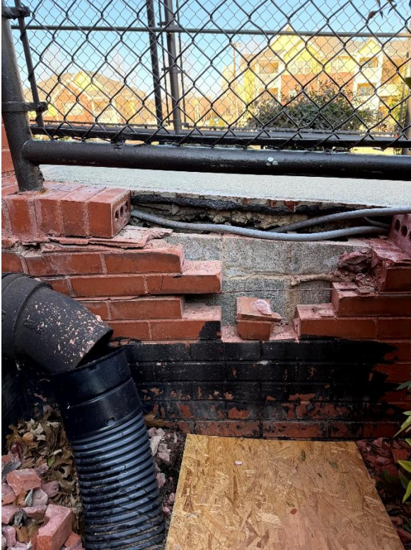
Photo 6 – South Ramp Wall
