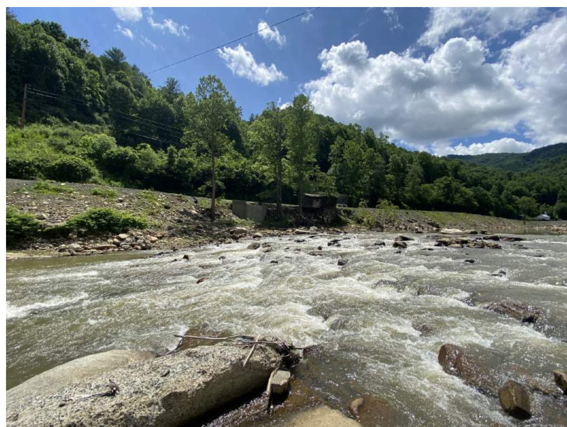
LOOKING UPSTREAM TOWARDS END BENT 2
