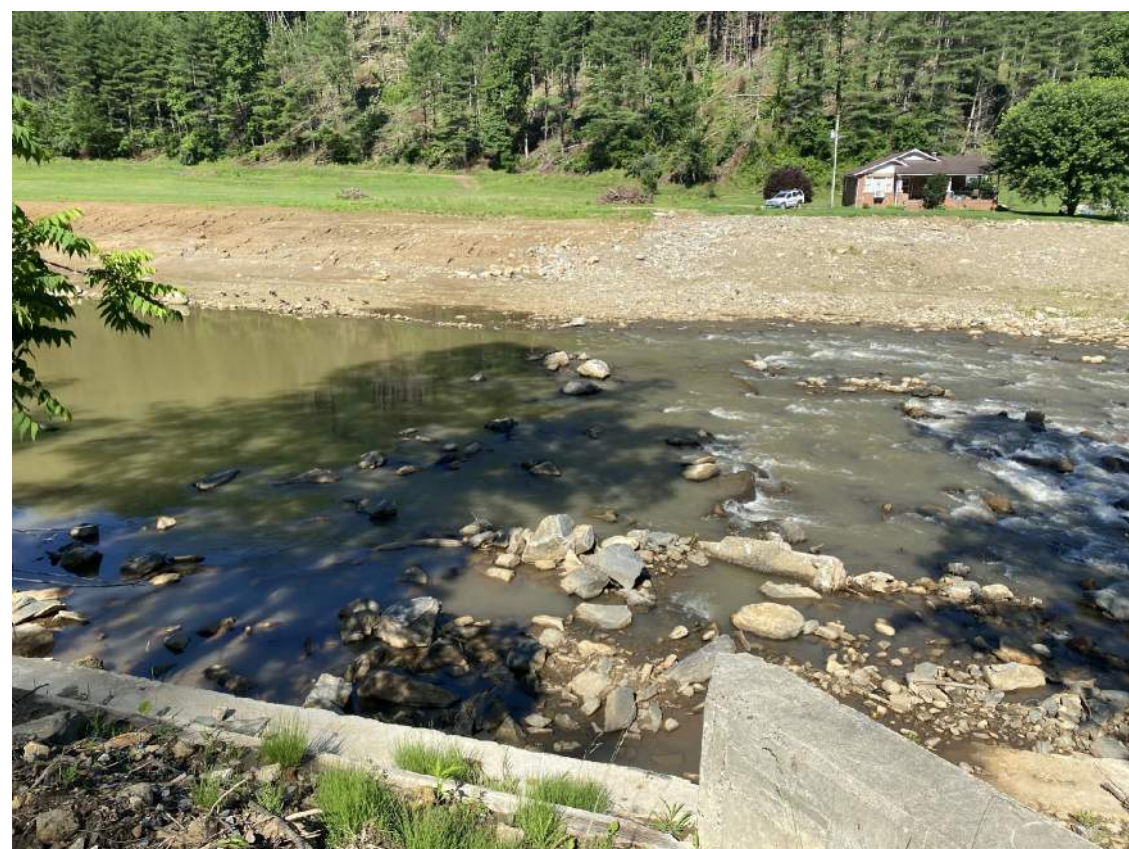
LOOKING WEST FROM END BENT 2
