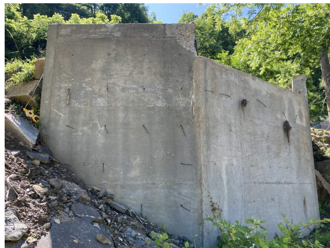
EXISTING END BENT 2
