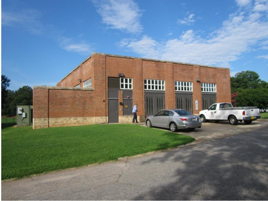
Photo: Chiller Plant
