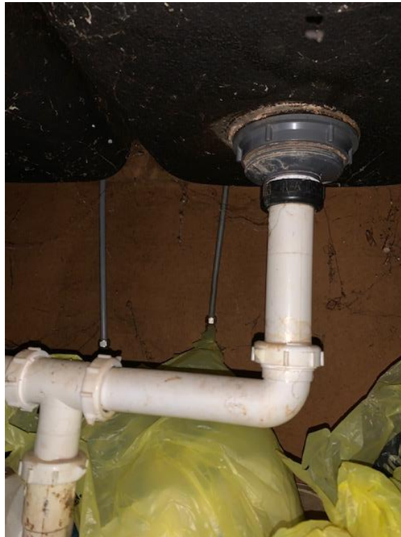
Asbestos-containing black sink mastic coating.
