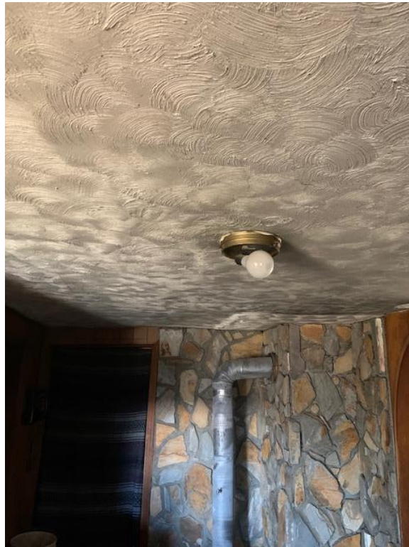
Typical view of asbestos-containing ceiling texture
