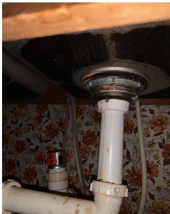
Asbestos-containing black sink mastic coating.
