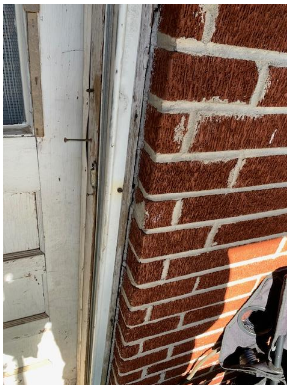
Asbestos-containing door/window caulk.
