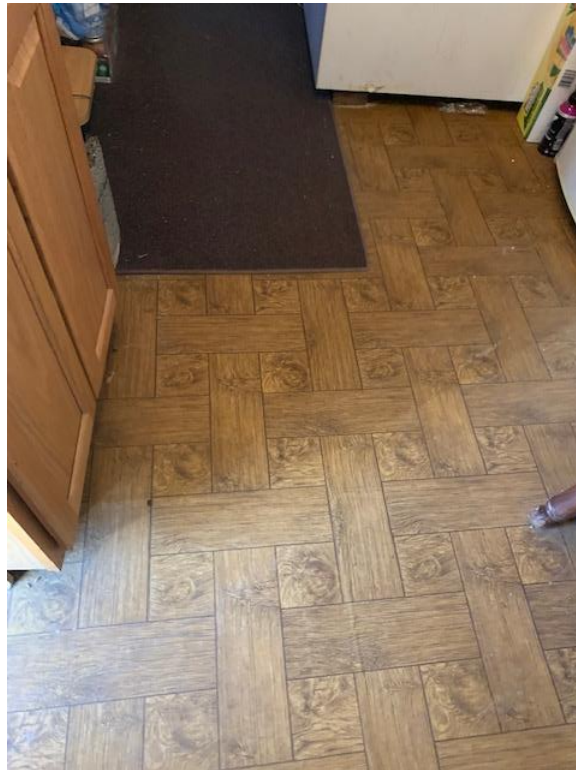
Asbestos-containing wood pattern vinyl sheet flooring.
