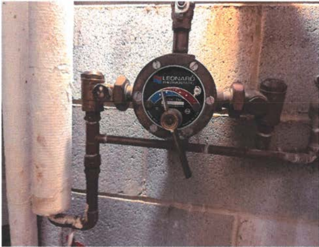
Photo 1 - Mixing Valve Assembly Photo 2 - Leonard Mixing Valve
