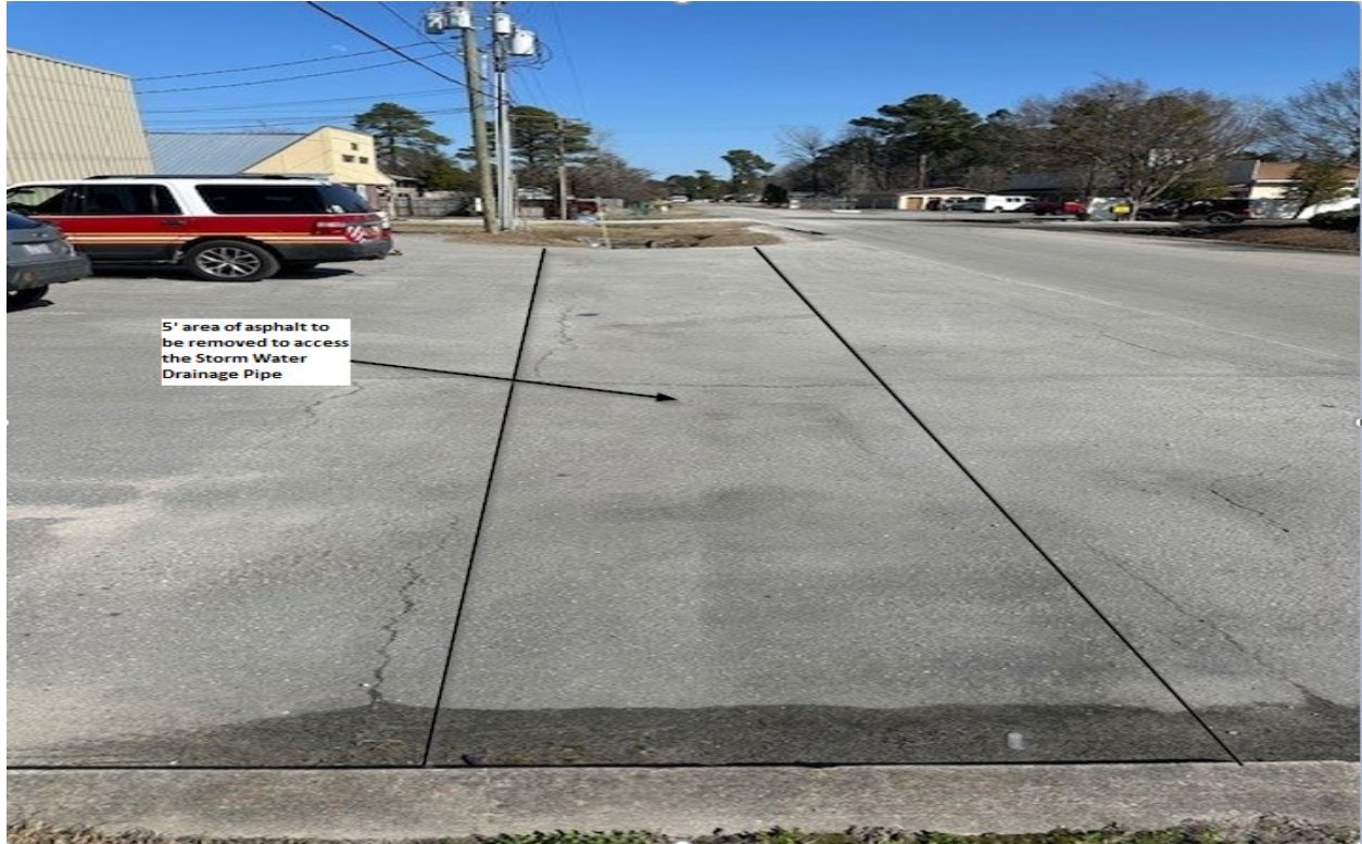
Figure 6: Asphalt Parking Lot and Driveway
