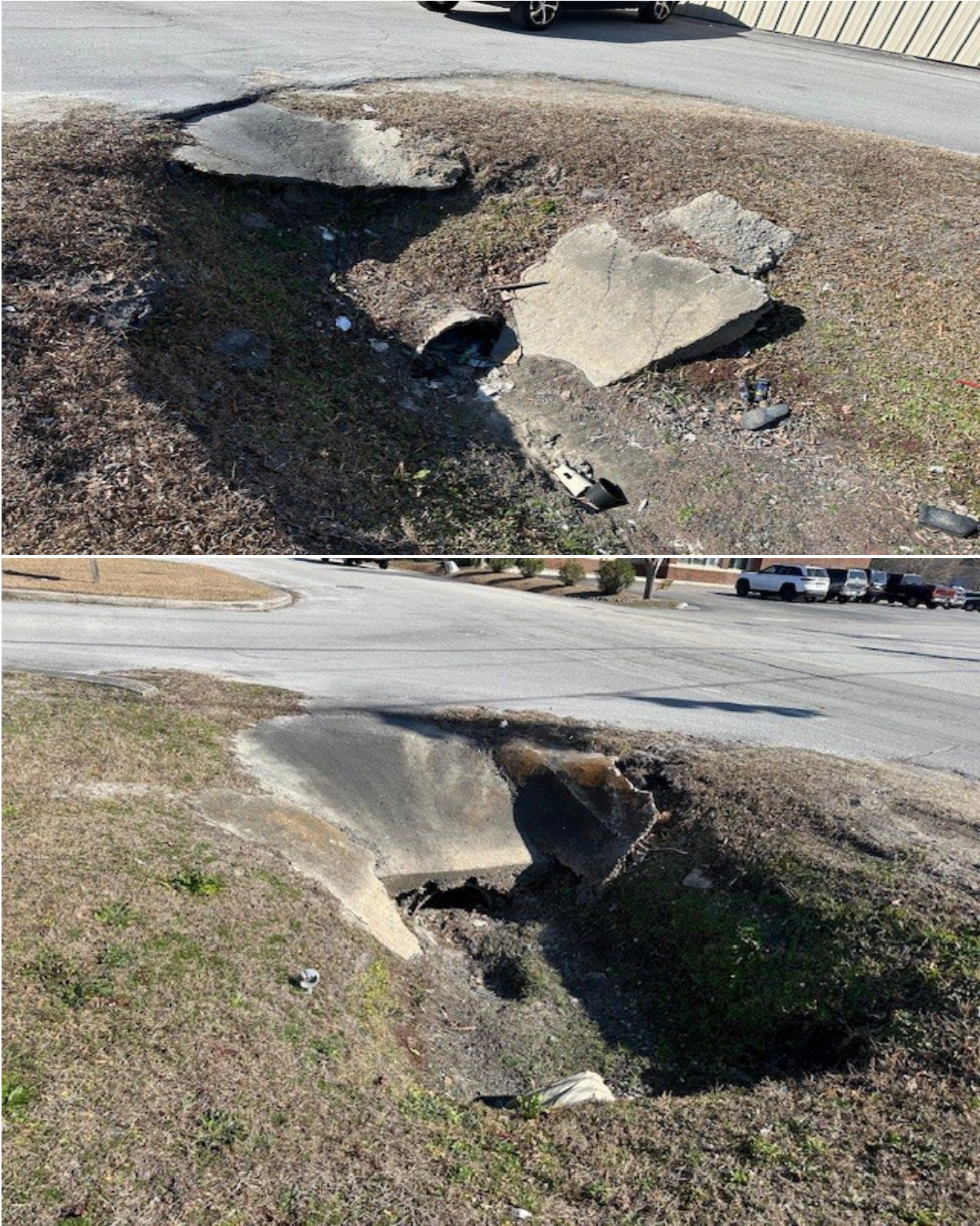
Figure 5: Images of Existing concrete flumes to be removed and replaced.
