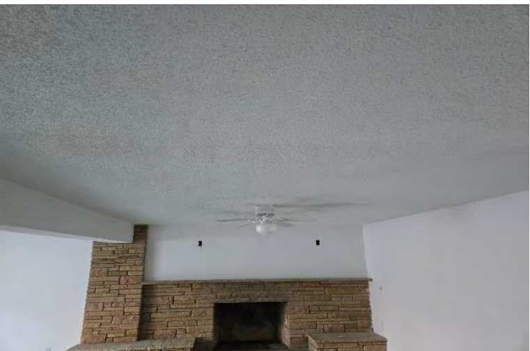
5. Basement Texture Ceiling. Sample A-10
