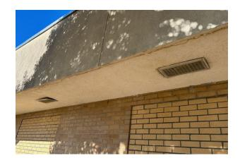
At the right rear of the gym, cover the exposed plywood on the soffit with metal and paint to match existing soffit as close as possible.
