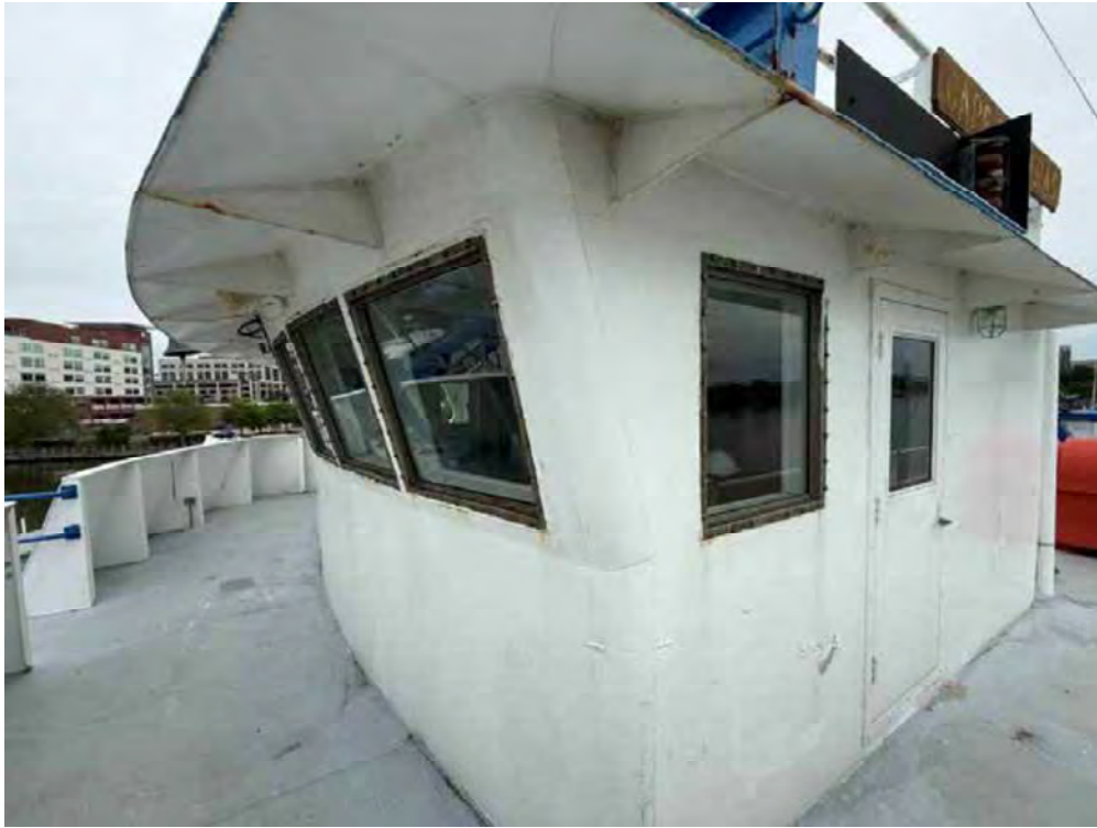
31. Bridge weather deck and house looking from port
