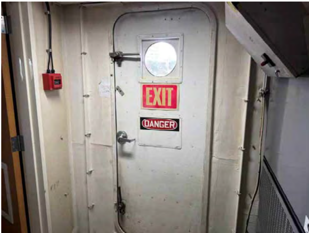
74. Typical watertight door access to weather decks
