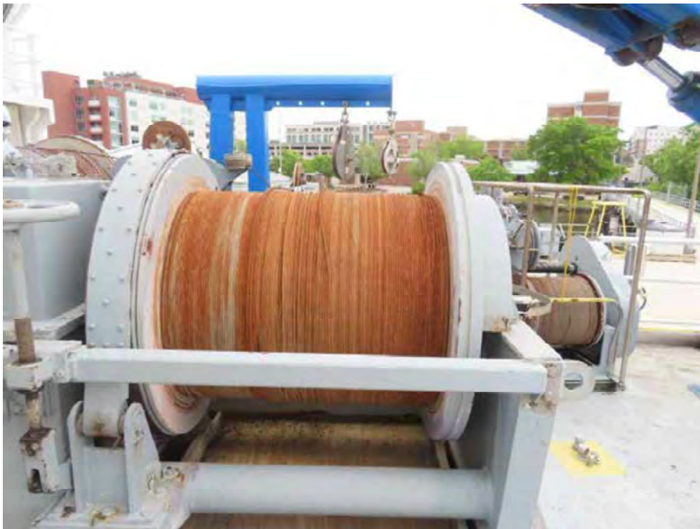
12. Winches for starboard side J-frame
