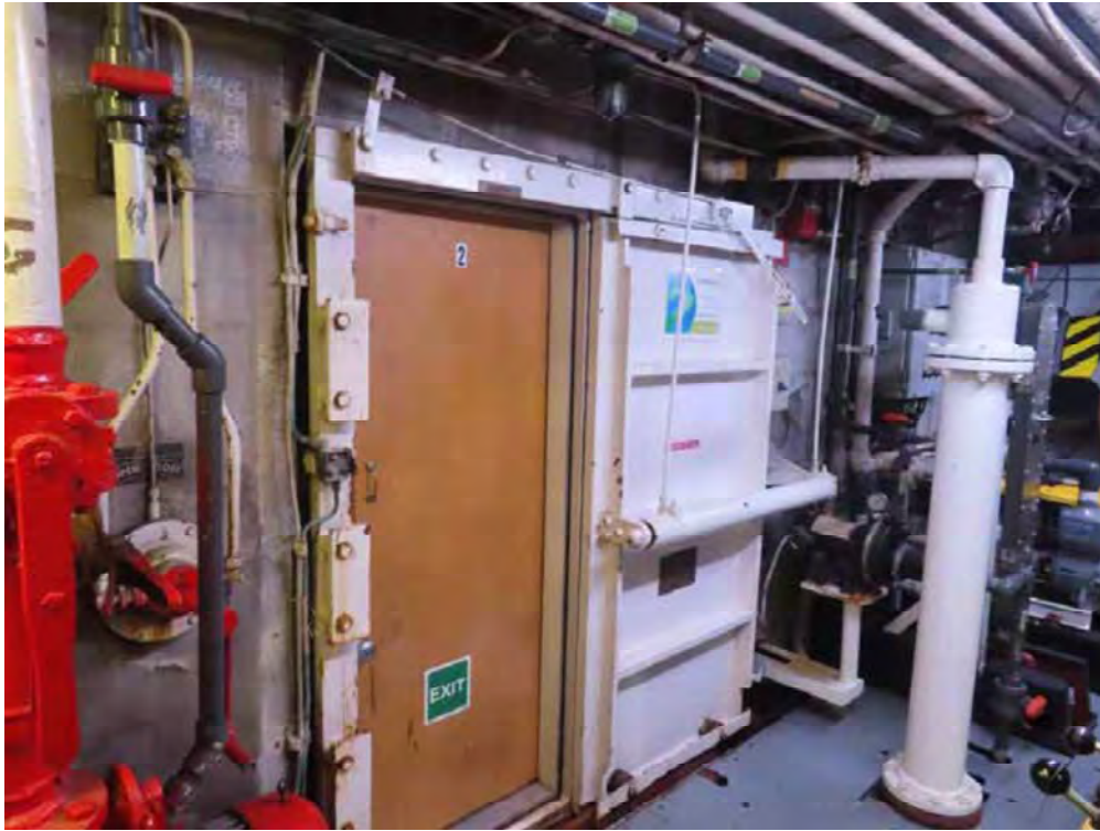
75. Watertight door to engine room
