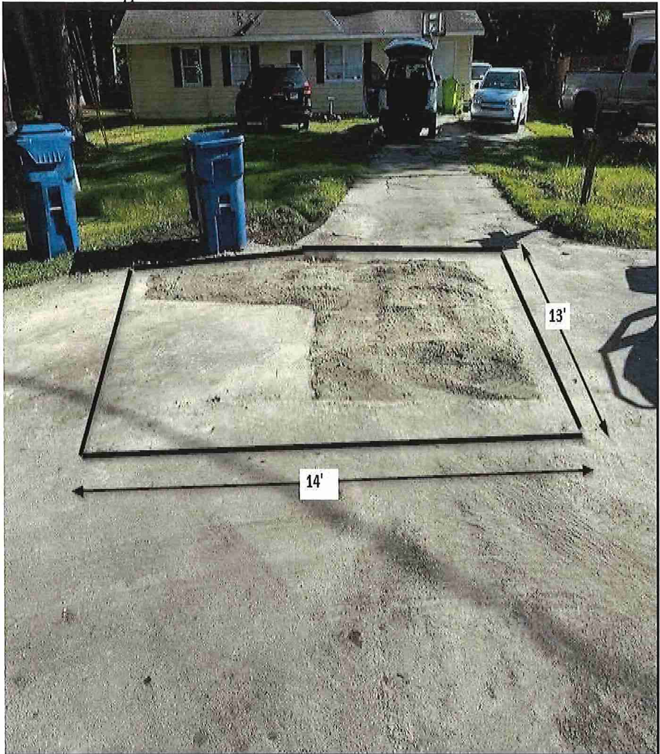
Figure 27: 508 Blarney / Area D / This area shall be cut square before repairing the utility cut. Measurements are approximate.
