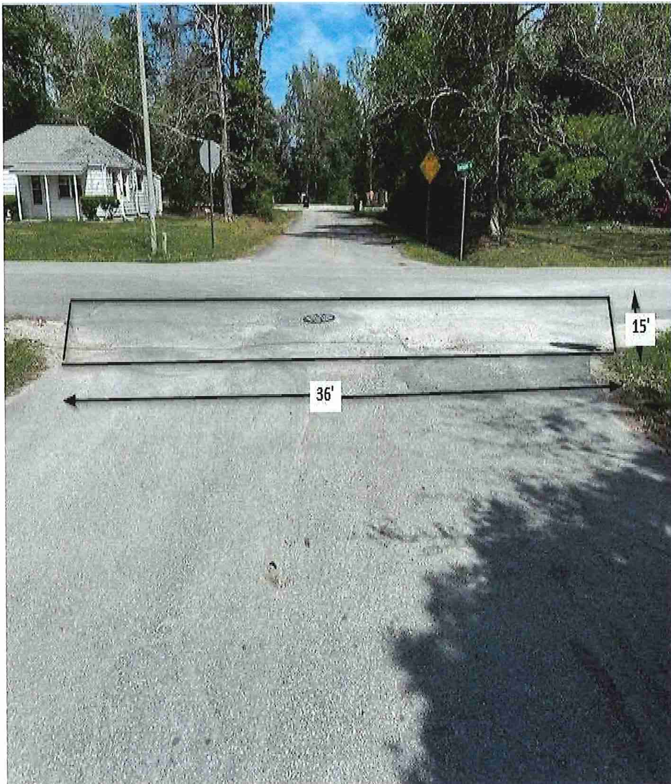
Figure 3: Fleetwood and Carolina / Area A / This area shall be cut square before repairing the utility cut. Measurements are approximate.
