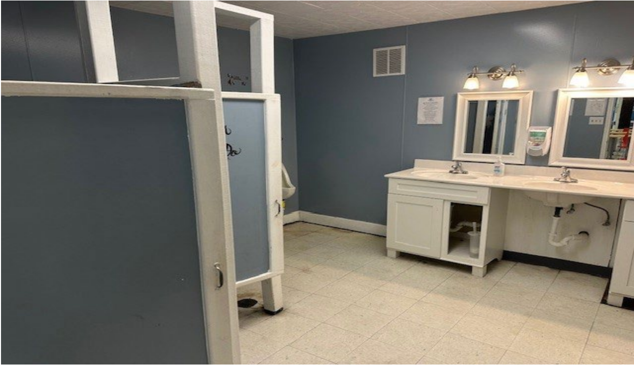
Figure 2: Images of the Boys' Bathroom.
