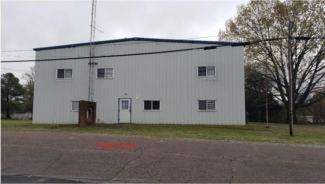
West Side Exterior
