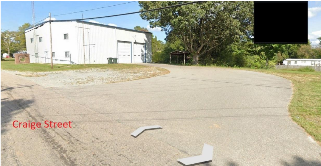
SW Corner Exterior / Existing Driveway
